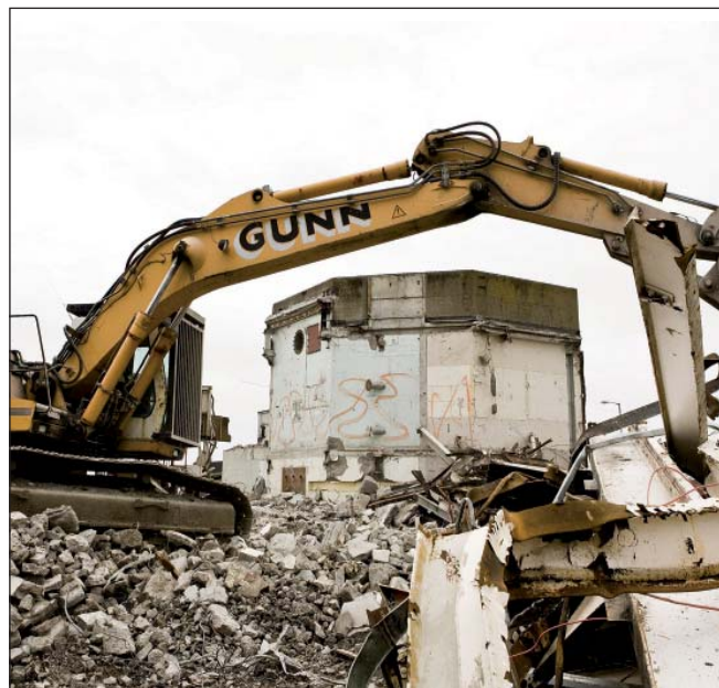
Demolition of nuclear facilities at Dounreay
